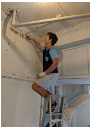
Finn, scraping away decades of paint in the maintenance room
